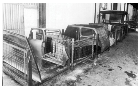
1,000 sets of Mini parts were made before the move over to Enfield.
